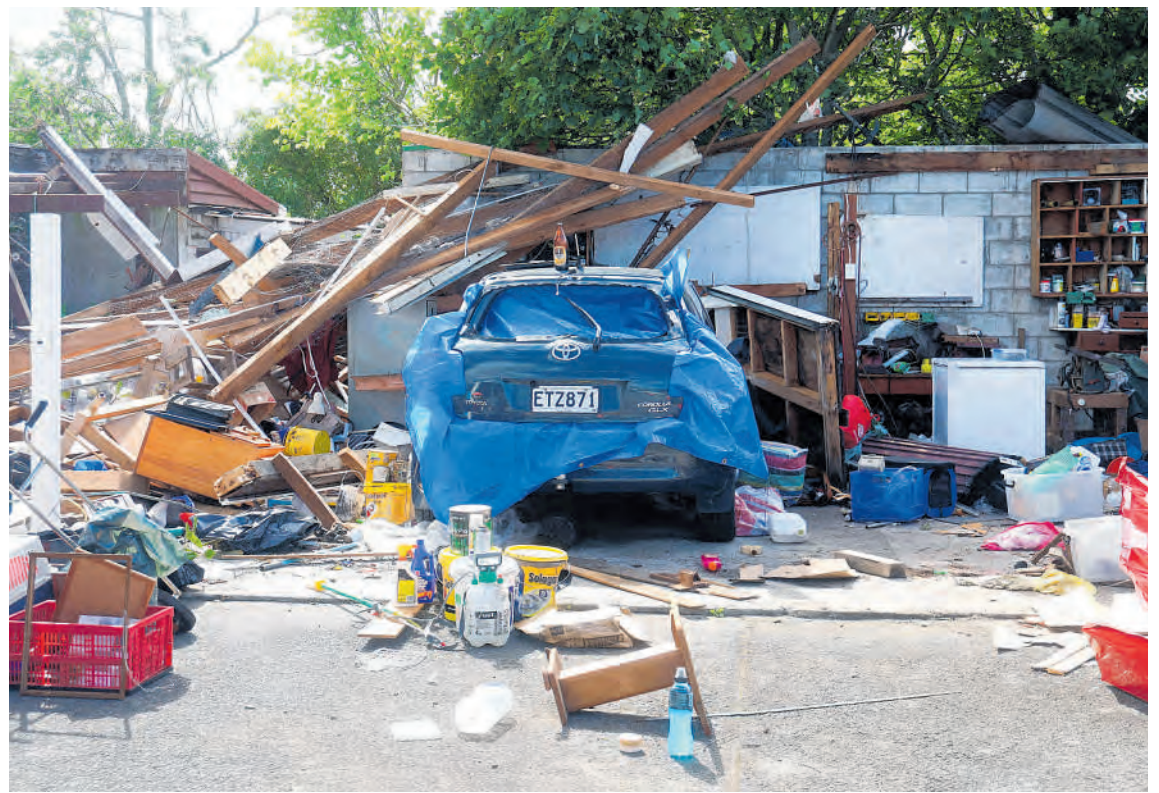
Properties in Lower Hutt were damaged when a severe thunderstorm hit the area on Tuesday.
