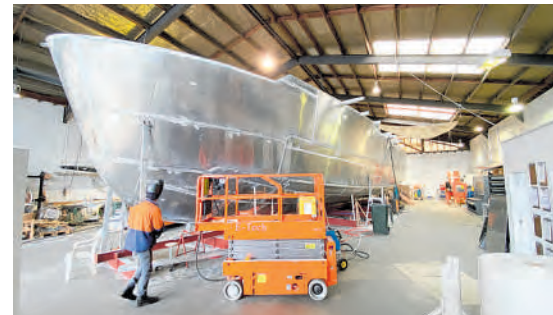
The aluminium luxury launch in the building stages at Northland Spares and Riggings.
